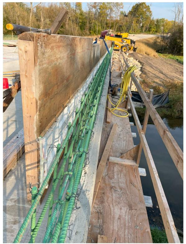
Parapet steel reinforcement and formwork with rock form liners.
