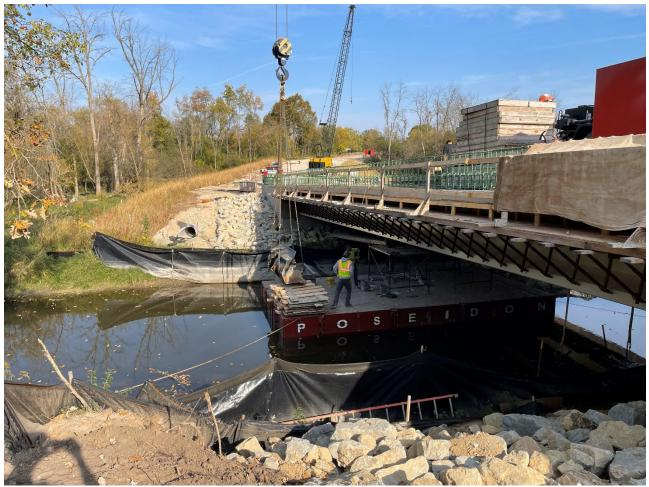
Stripping underside formwork on barge.
