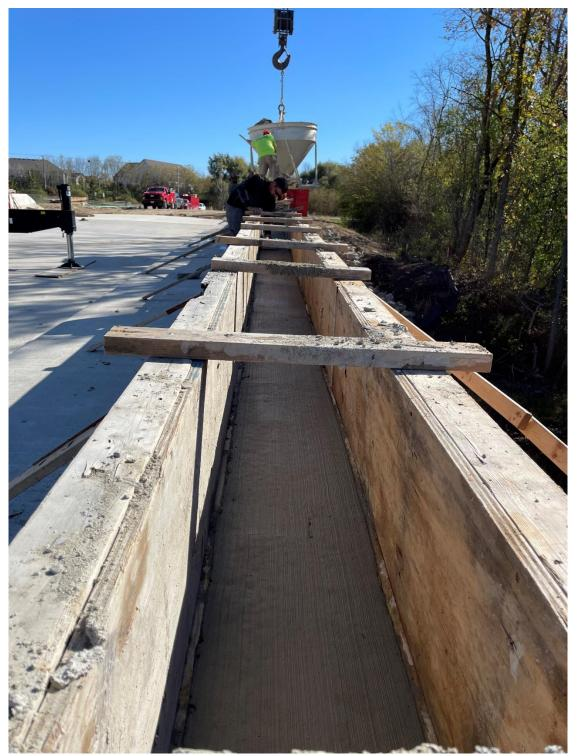
Parapet freshly poured in formwork.
